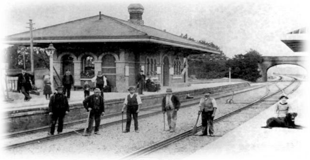
Figure 1; Mortimer railway station
