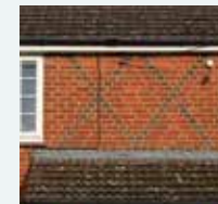
Diaper pattern brickwork
