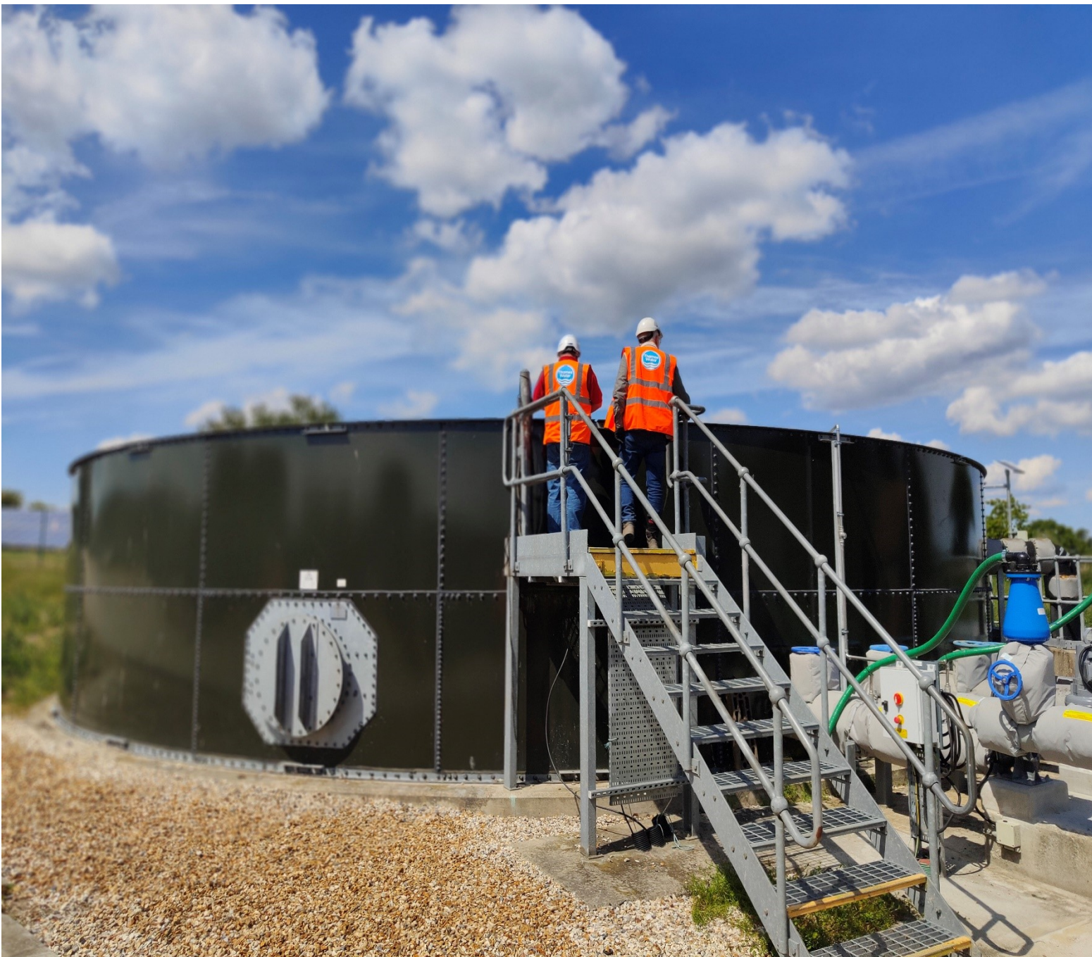
The storm discharge storage tank. When storage is full and incoming flow is greater than the rate of treatment sewage is diverted to this tank. When possible it is returned to the incoming flow. New pumps will speed this return.
