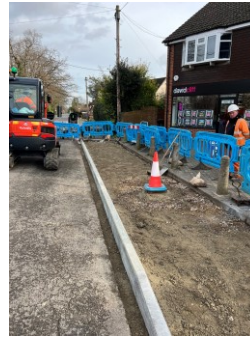
Remedial work starts
