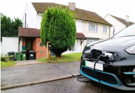
Cross-pavement cable trial
