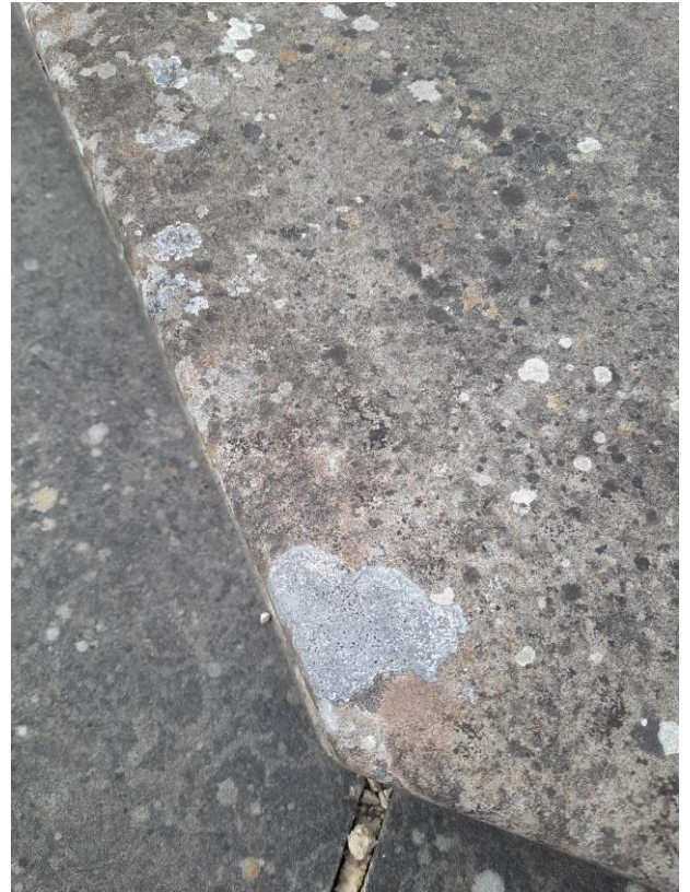
Figure 8: Lichen and broken mortar on base steps
