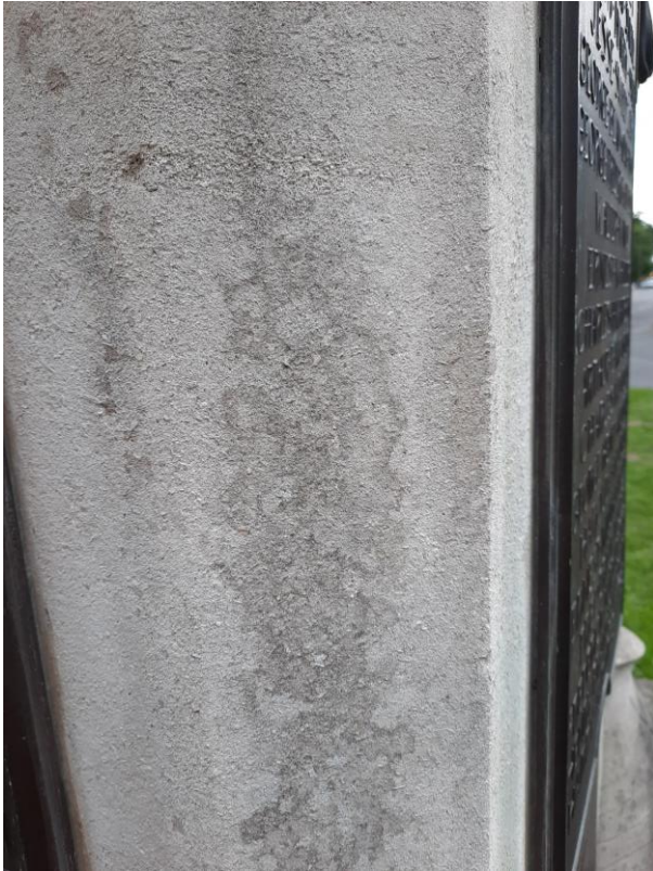
Figure 5: build up on stone surface
