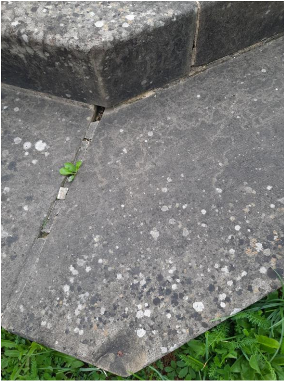
Figure 1: lichen and stains on steps at base
