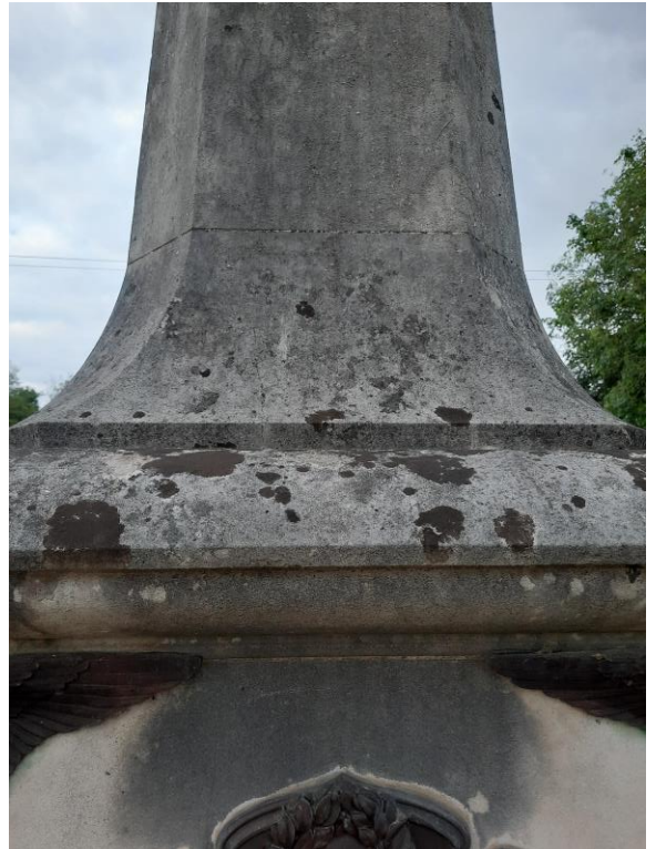
Figure 2: lichen and stains on plinth
