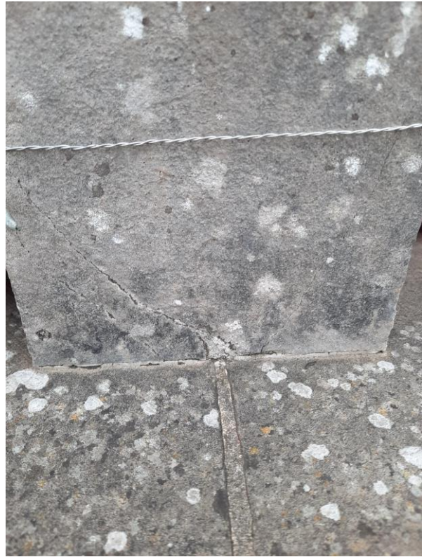
Figure 7: Lichen and fractures on base
