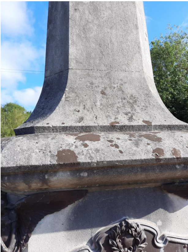
Figure 10: deposits and cracks
